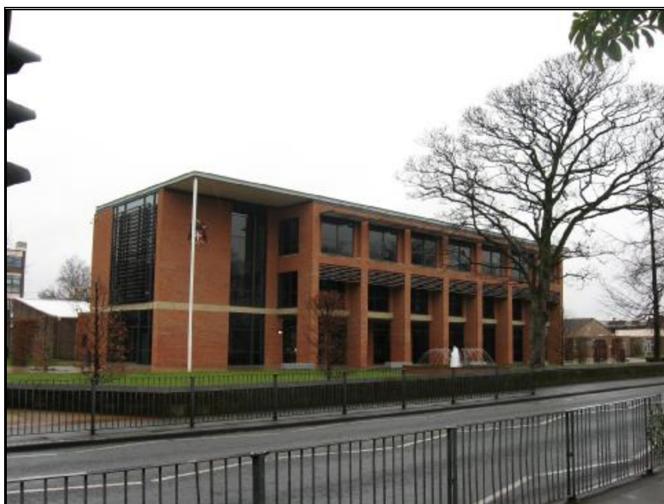
Picture 1 A view down Taggart Avenue, April 2009, showing the Foundation Building
